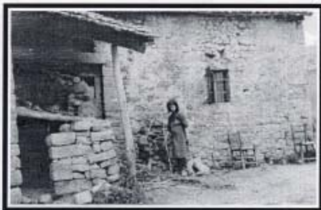
Typical Apennine farm house on Sprilla Road.
