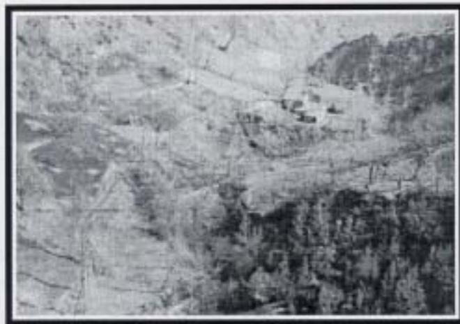
A view down the valley from midway across the Campidello - Castellaccio cableway.
