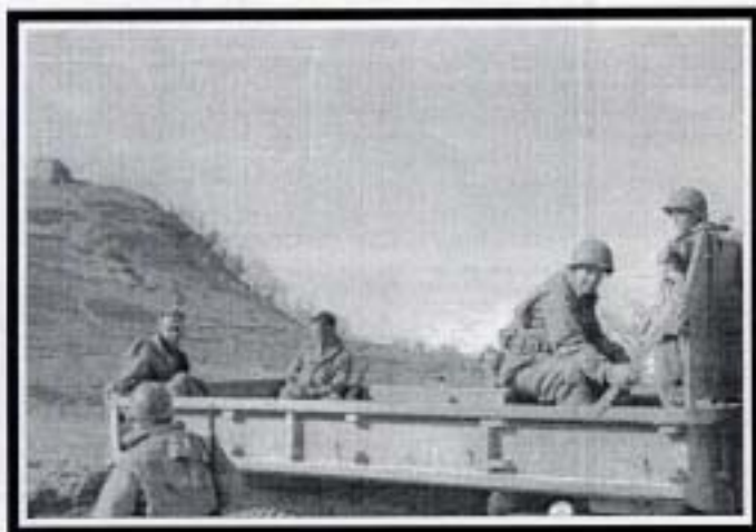
Loading up at Gaggio Montana for a day's work on the Sprilla Road rebuild project.
