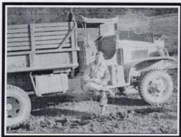
Lt. John Sheahan, 1st Platoon's boss, checks out the morning Blizzard on the Sprilla Road job.
