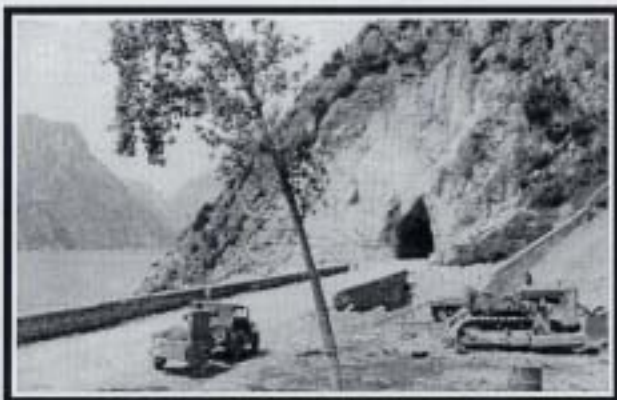
After it was cleared.
