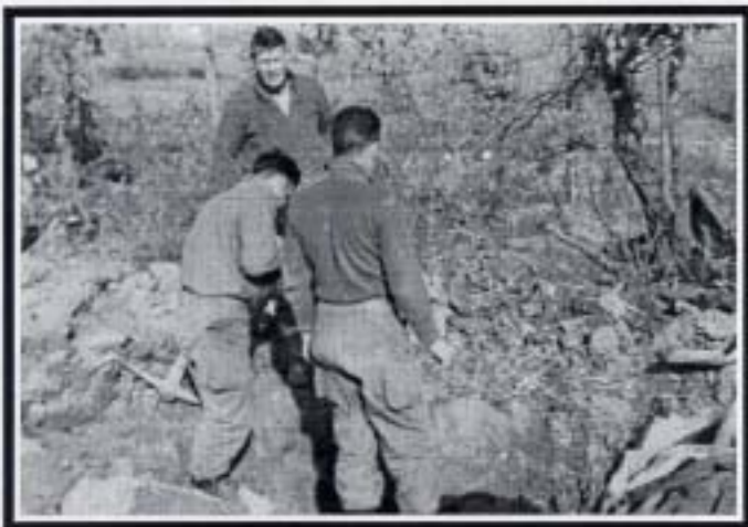
Floyd Grigory checks out the design of this dug-out.
