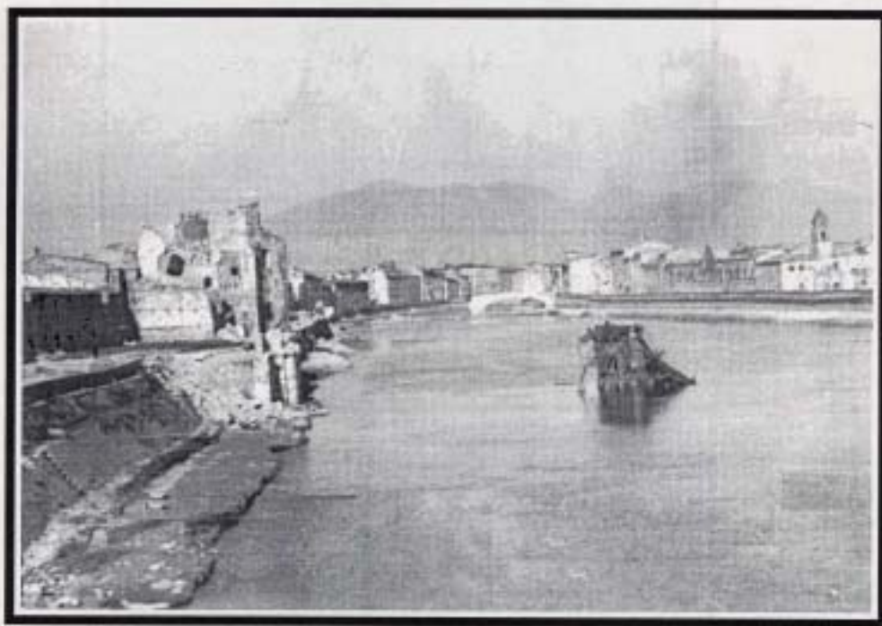
Total destruction along the Arno River in Florence where the Germans mounted a desperate defense in the late fall of 1944.
