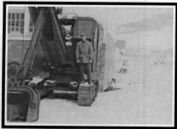
Dick Sweet checks out the 226th's power shovel.
