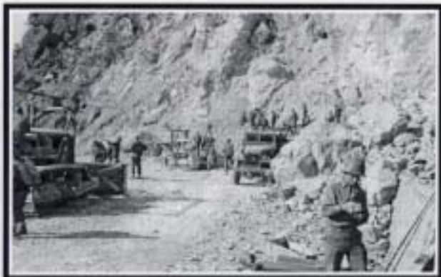
Tunnel # 1 on the east shore of Lake Garda, blown by retreating Germans, before it was cleared by Company D.
